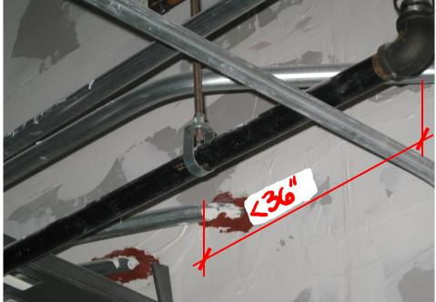
Support of straight run, on a system that does not exceed 100psi system.
