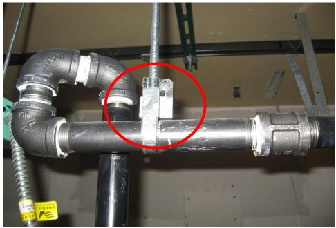
Uplift Clip on an arm over on a system that exceeds 100psi system.
